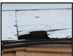
Moisture has penetrated the siding in areas causing rot. All rotted siding should be replaced or repaired with a patching material designed for wood repair (1C.06).
