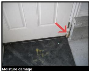
Hardware operational, Damage noted at the lower trim of door opening. Water seepage appears to be occurring.
