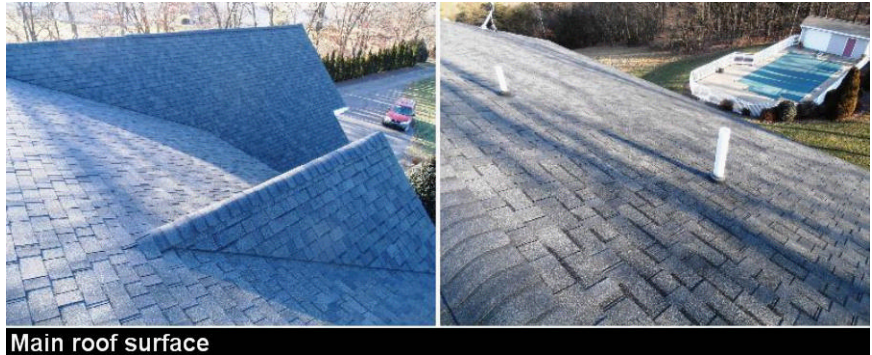
Main roof surface
