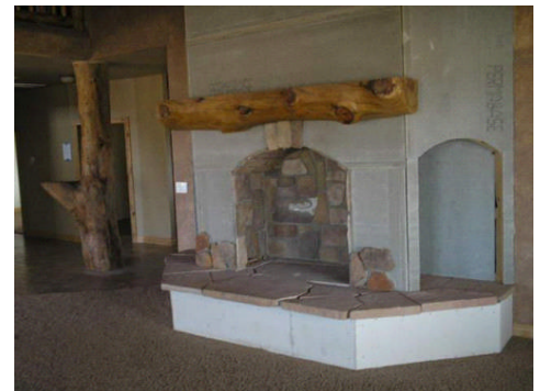
Fireplace not complete
