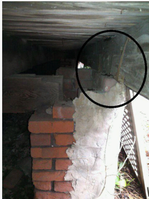
Wood and posts hardly supported.
