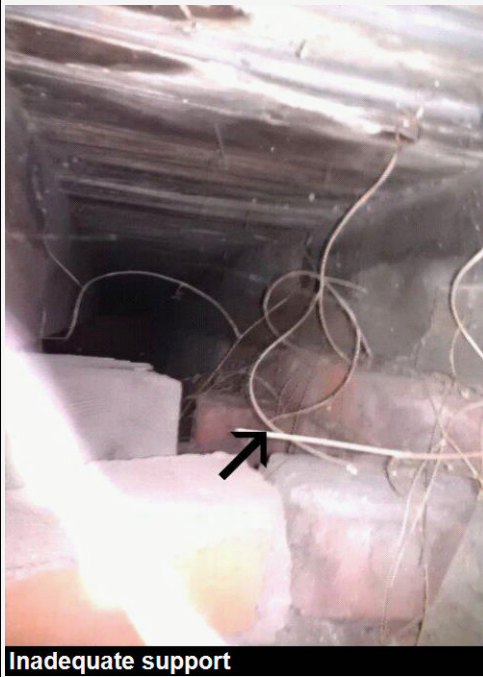
Loose brick at pier
