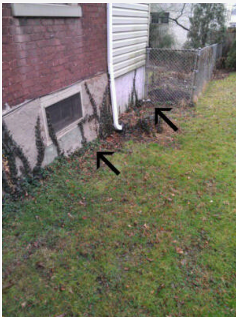
Negative pitch towards foundation walls
