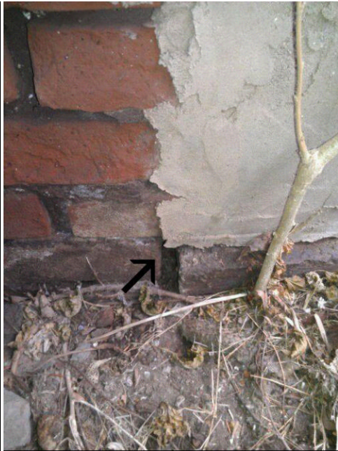
Loose brick at pier
