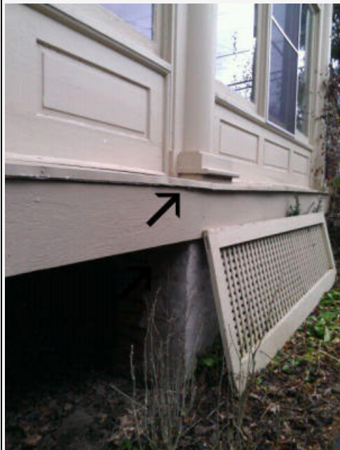
Wood and posts hardly supported.
