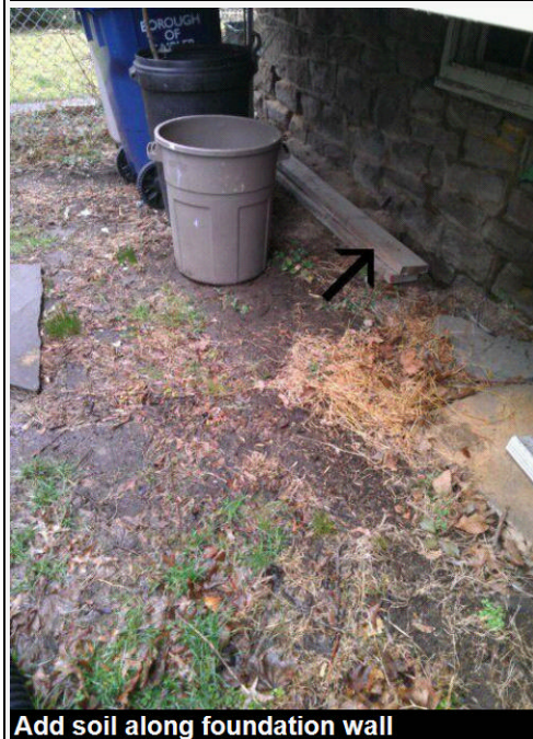
Negative pitch towards foundation walls
