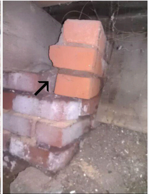
Loose brick along front columns
