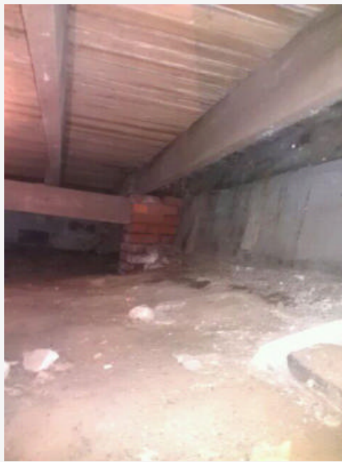
Moisture damage and settlement
