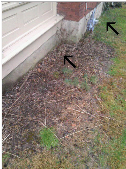
Negative pitch towards foundation walls
