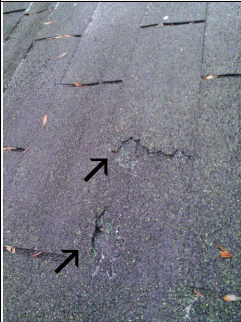
Deteriorated shingles
