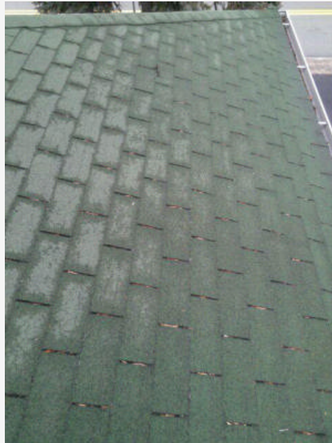
Water stains / evidence of leakage.
