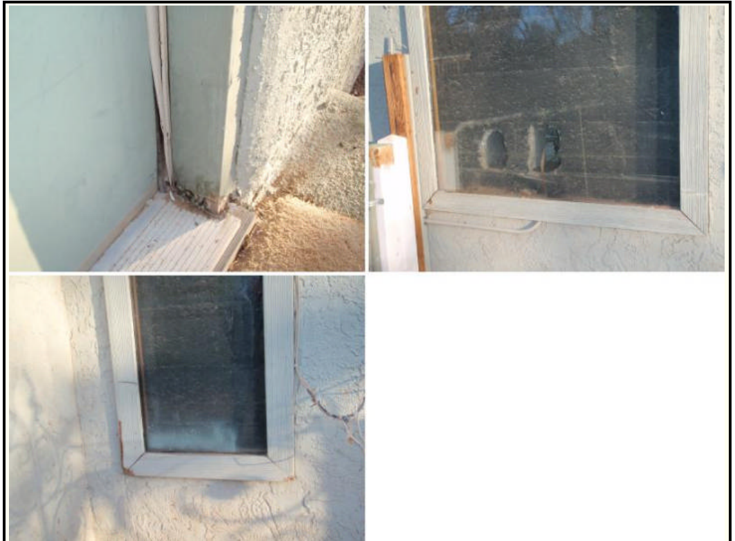
Refinish trim on the south side.
