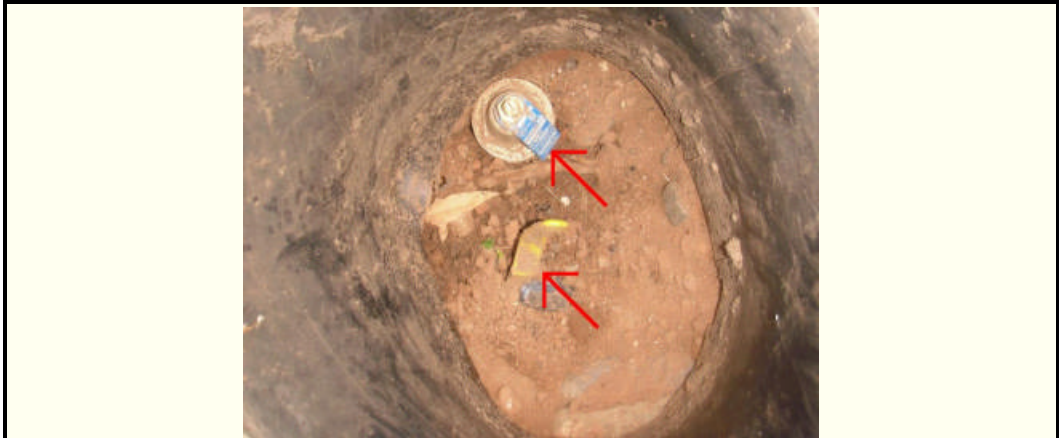
Main water valve and pressure regulator.
