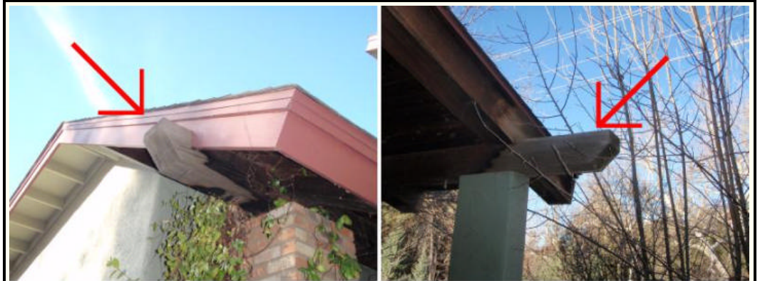
Consider flashing caps on the exposed beam ends.
